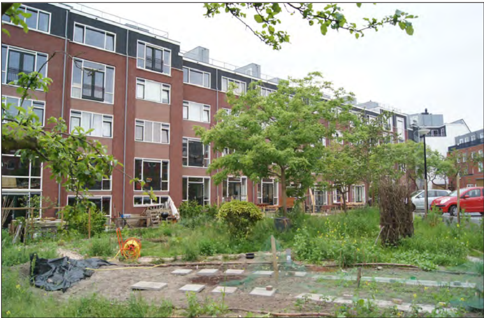
Fig. 3. Renovation by means of self-built housing and co-housing.
